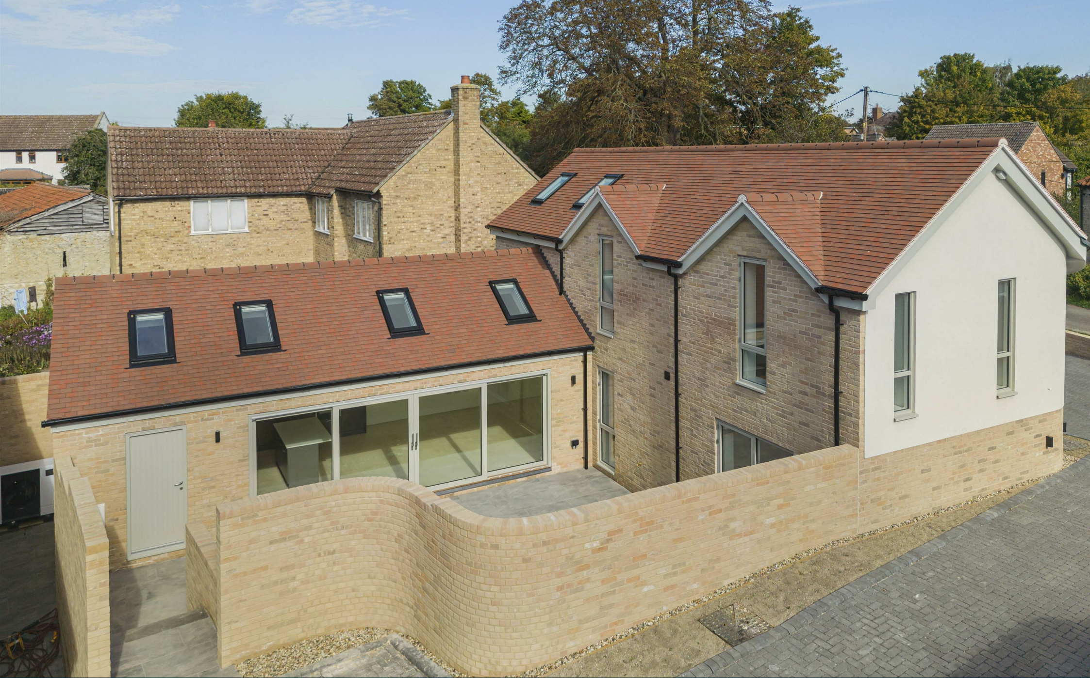
Pudding House, Mill Lane, Burwell CB25 0HJ
